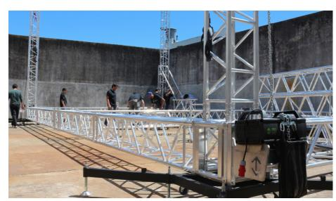
It is very important that the hoist hook and lift hook run in line with the direction of forces. It is not permitted to have the lift chain run with a fleet angle into the chain hoist nor to attach the load hook at an angle, for example to the sleeve block, because this will exert a side load on the hoist housing.
